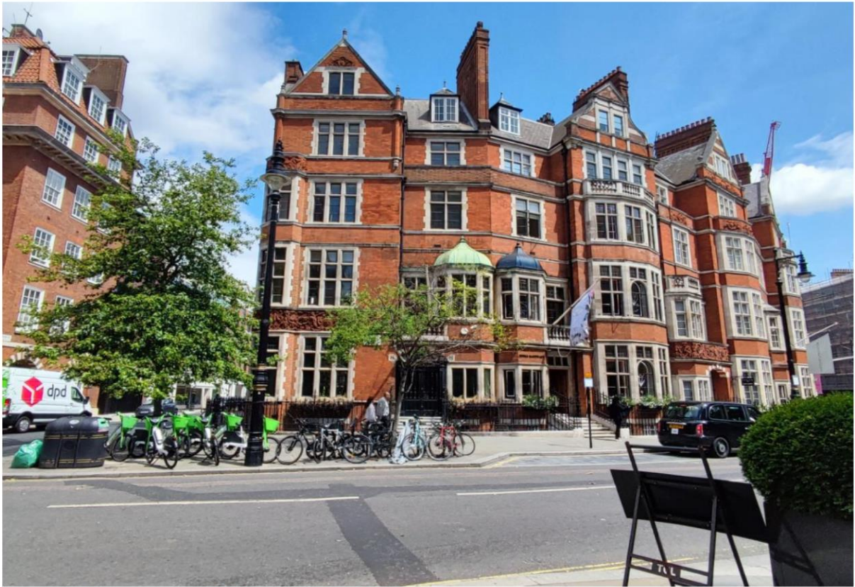
Figure 1: View of front of building. Note there is one cab in rank to the right of image
