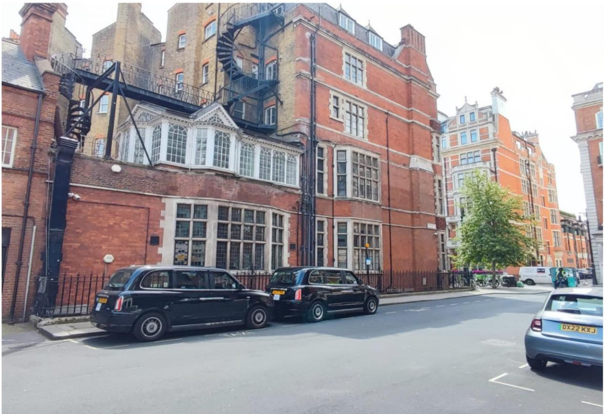
Figure 2: View of side of building with feeder cab rank for up to five cabs
